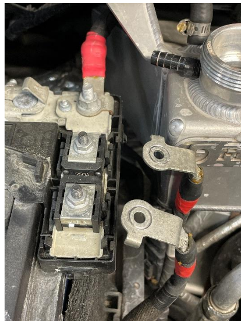
Figure 9: Removal of each auxiliary cable from the positive terminal.
