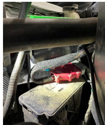
Figure 9: Routing of Tapshifter harness.
