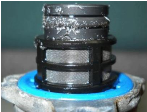
EXAMPLE OF CONTAMINATION FROM CATESTROPHIC PUMP FAILURE
